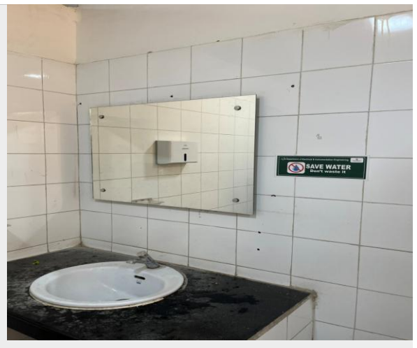
Gents Washroom, BC-Block, Ground
